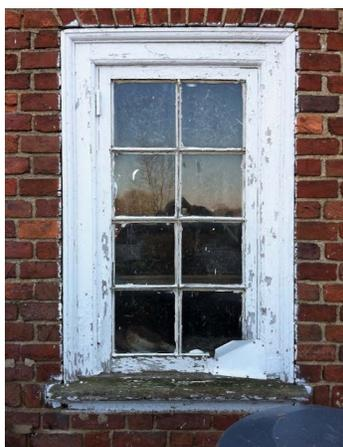
Windows are often referred to as the "eyes" of a building and are a character-defining feature that provides scale, profile and composition to a facade. Many of Stroudsburg's windows are of the double hung sash variety, a window style dating back over three centuries in America.
