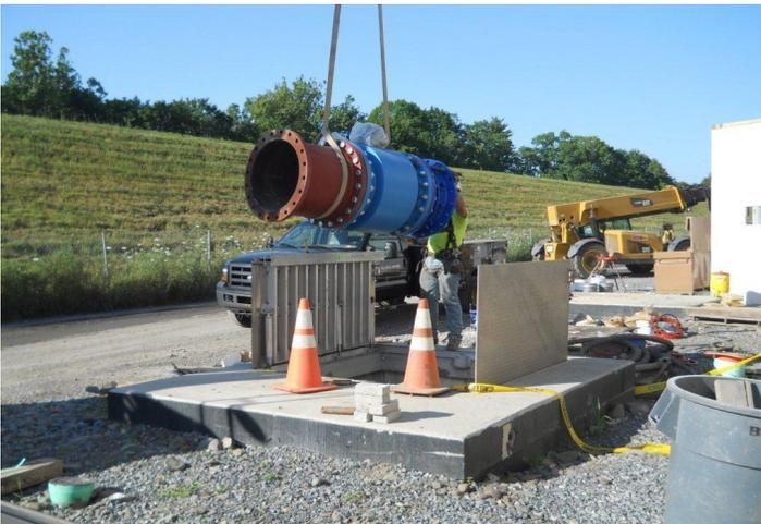
**Installation of a flow meter as part of the Plant improvements, with the levee shown in the background.**
